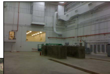
New Experimental Hall D awaiting equipment installation
